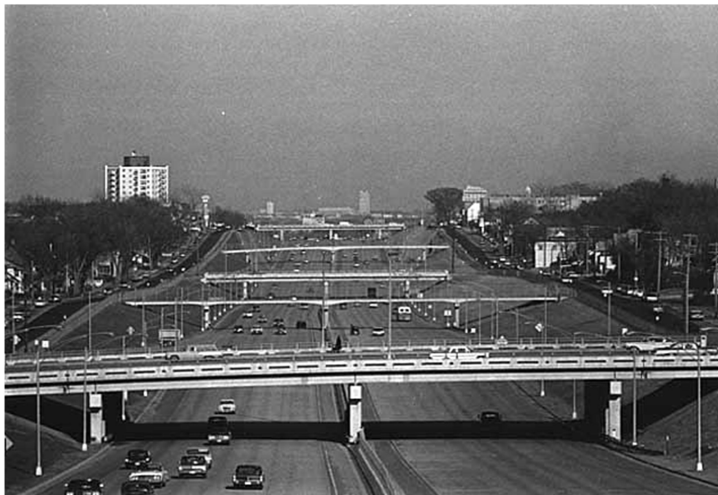
On Dec. 9, 1968, a new 11-mile segment of Interstate 94, linking downtown Minneapolis with downtown St. Paul, opened for the first time.
